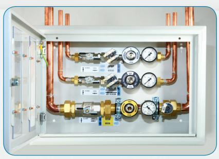
Their function is to allow, thanks to the built-in ball valves, the exclusion or the passage of the medical gases in a service or area and to define this area from the rest of the network. Downstream each valve for compressed gas it is installed one pressure switch and a specific gas coded emergency terminal unit.
